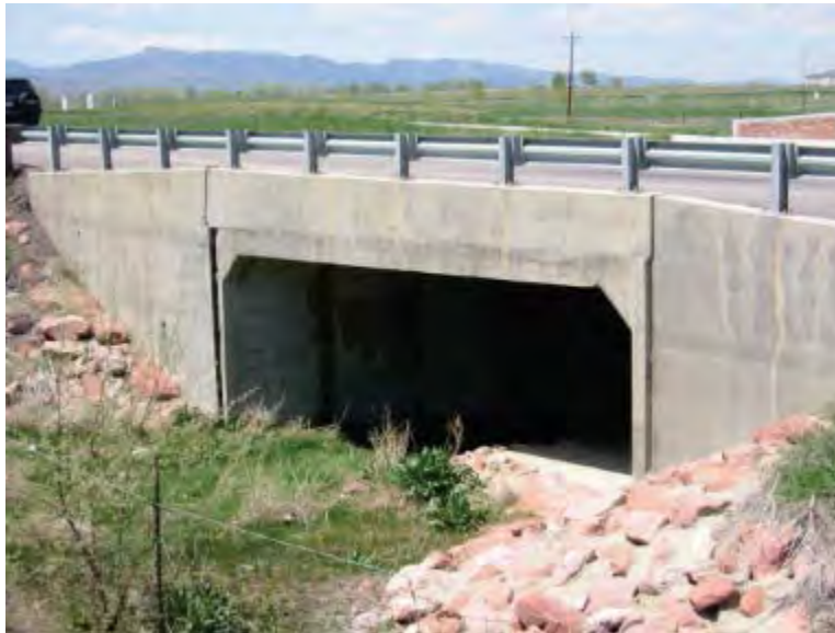
Figure 7-2 Concrete box culvert (from FHWA, 2012)
